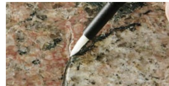
Apply primer (for bonding)
