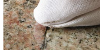
Clean the preparation
