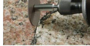
Prepare the damaged surface
